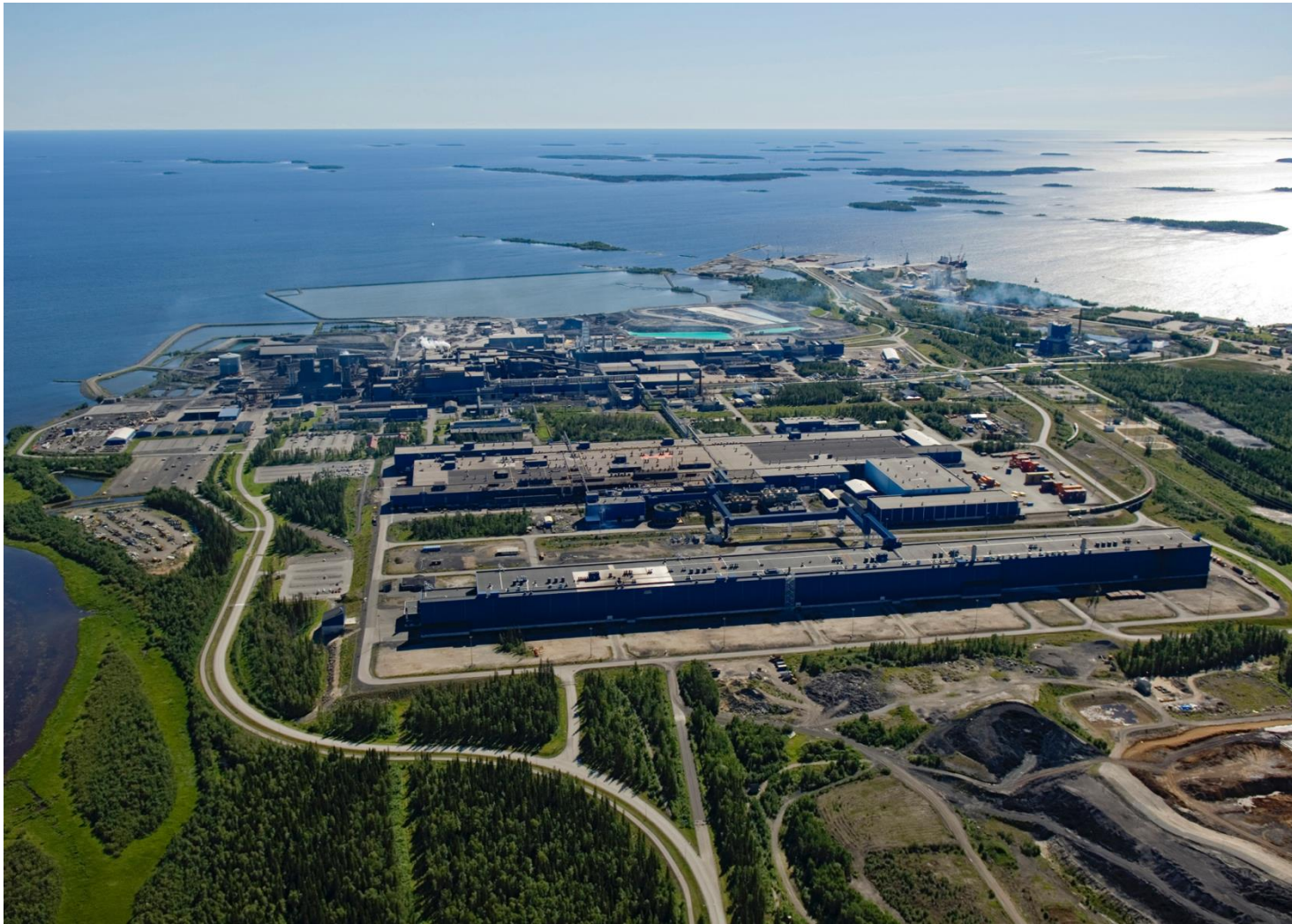
Outokumpu's site in Tornio (stainless steel production facility)
